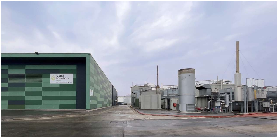
East London Biogas plant for which HZI will deliver new equipment ©Bio Capital Ltd.
