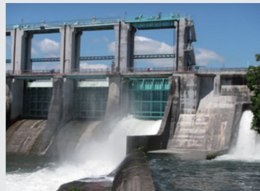
Gate in Ishibane Dam (Iwate Prefecture)
