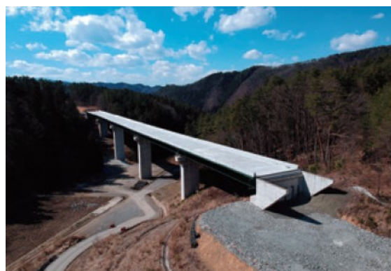
Mihari Viaduct of Chubu-Jukan Expressway for Chubu Regional Development Bureau
