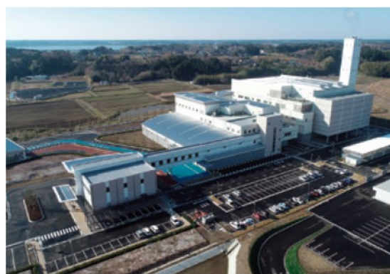
Waste Treatment Plant in Mito City (known as "Ecommit") (Ibaraki Prefecture)
