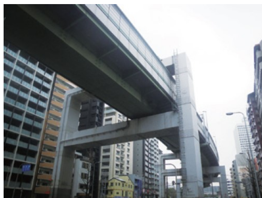
Near Awaza Junction, Hanshin Expressway
