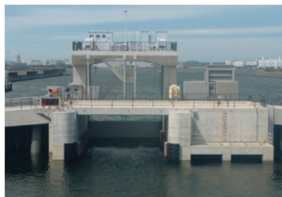
Hydraulic gate in Sea Forest Waterway for Tokyo
