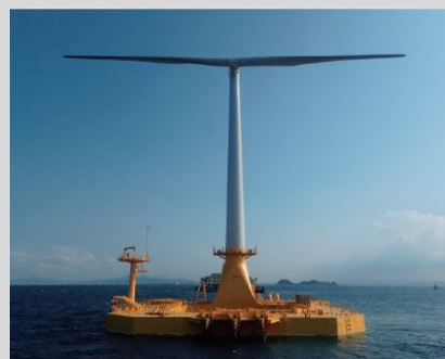
Floating offshore windfarm system demonstrator
