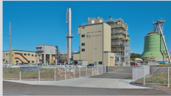
Woody biomass power plant
