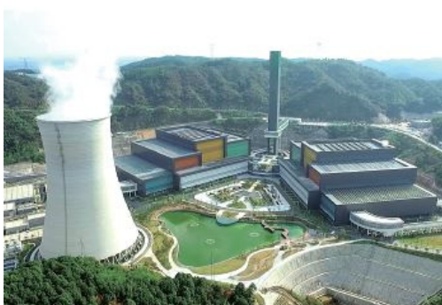
EfW plant in Changsha City, China (Phase 1)
