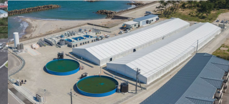
Onshore Aquaculture Plant (Water Treatment System)
