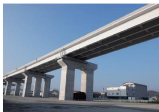
Tsuda Viaduct for Shikoku Regional Development Bureau
