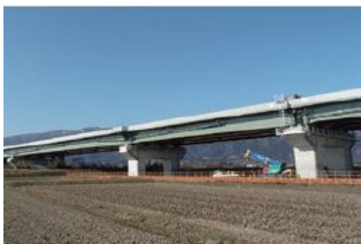
Yogegawa Elevated Bridge
