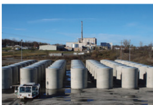
Nuclear spent fuels storage vessels (56 canisters) for the U.S. Department of Energy's project to close down reprocessing plants
