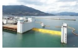
● Seabed system flap-gate seawall to safeguard against flood disasters
