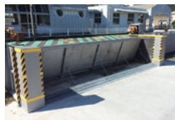
● Flap-gate type seawall against flood disaster
