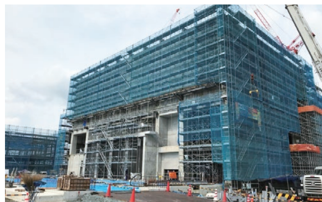
EfW Plant for Kikuchi Environmental Preservation Association
