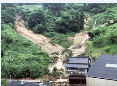
Landslide near the plant
