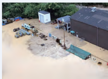
Flooding and mudflows within the plant grounds
