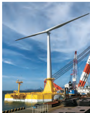
Left: barge-type floating body of an offshore windfarm system (June 2018, Sakai Works)
