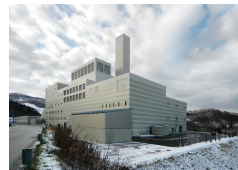
Waste to Energy plant, Otaru City
