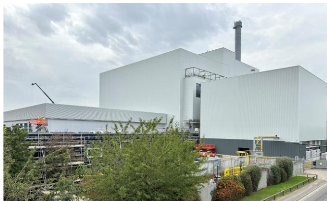
Waste to Energy plant, Slough, UK (Oct. 2023)
