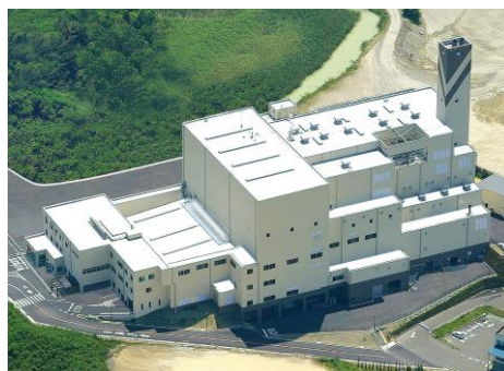
Waste to Energy plant, Jo-yo City
