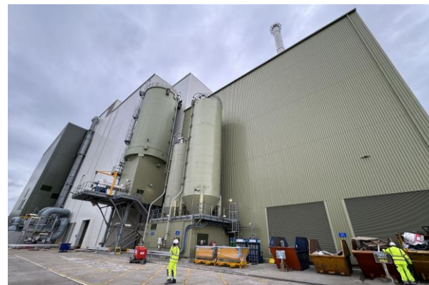
Waste to Energy plant, Earls Gate, UK (Oct. 2023)
