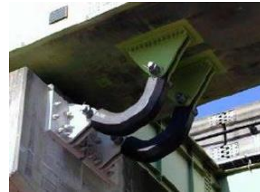
Bridge girder connection with rubber-coated chain
