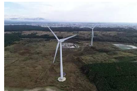
Omagari Wind Power Station currently in operation (Akita city)
