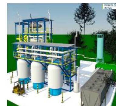
Image of Methanation facility (Synthetic methane production: 1,200 Nm 3 /h)
