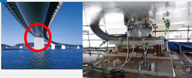
Measurement of bearing part and bridge pier displacement
