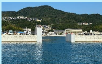
Bridges, Hydraulic gates
