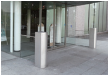
The "neo RiSe" seawall installed at the entrance to the Company's head office
