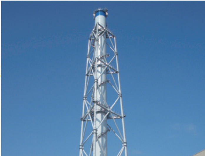
Steel-stack for Kashima Kyodo Electric Power Co.
