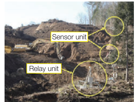
Landslide monitoring system employing GPS high-precision positioning devices
