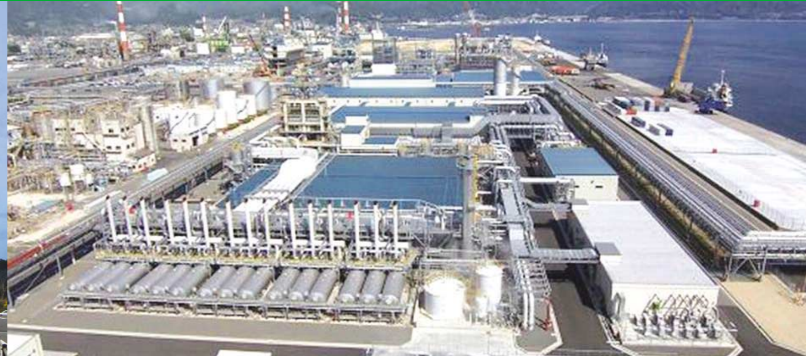
Acetate tow manufacturing plant
