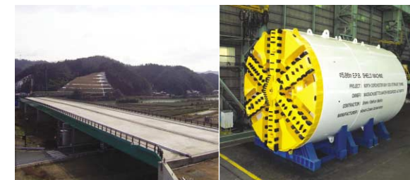
Construction of the upper section of Okawa bridge for Kyoto Prefecture Shield tunneling machine for America
