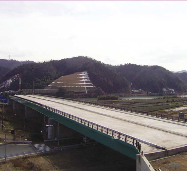
Construction of the upper section of Okawa bridge for Kyoto Prefecture
