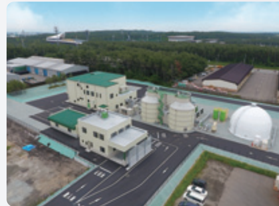
Akita Biogas Power Station
