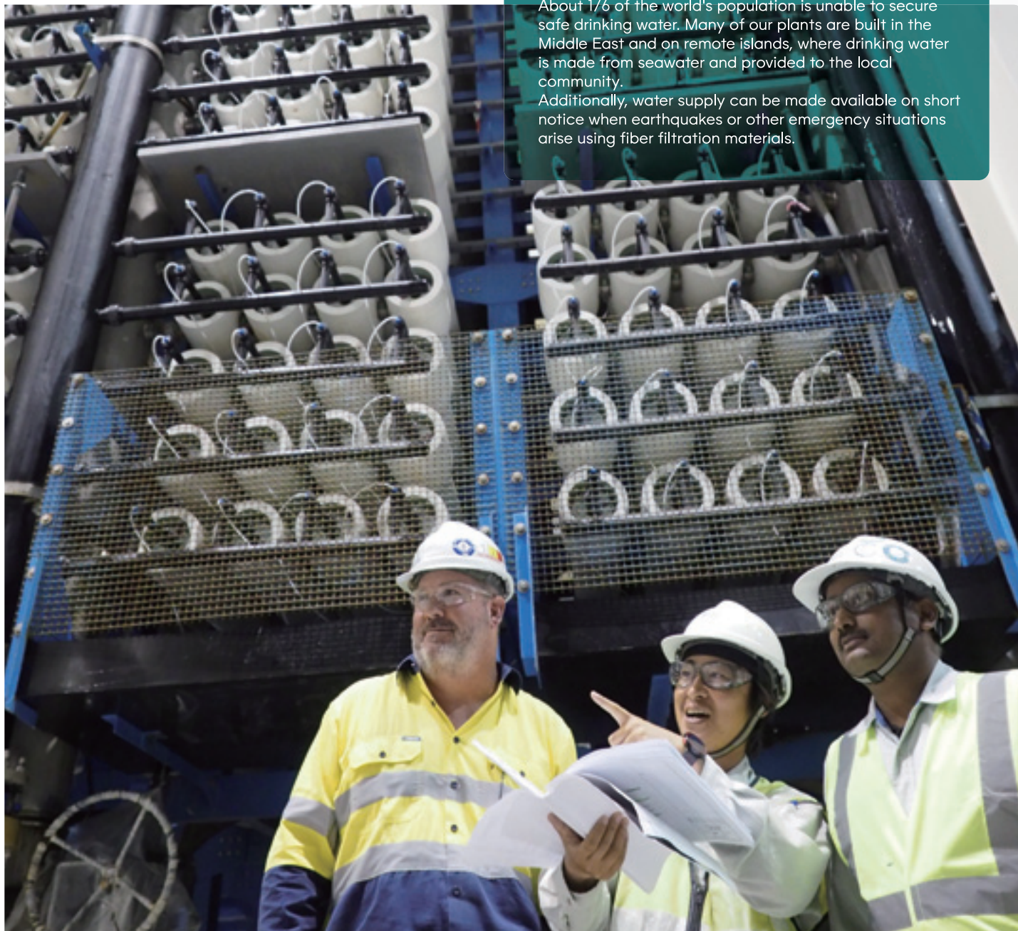
RO Seawater Desalination Plant (Qatar)
