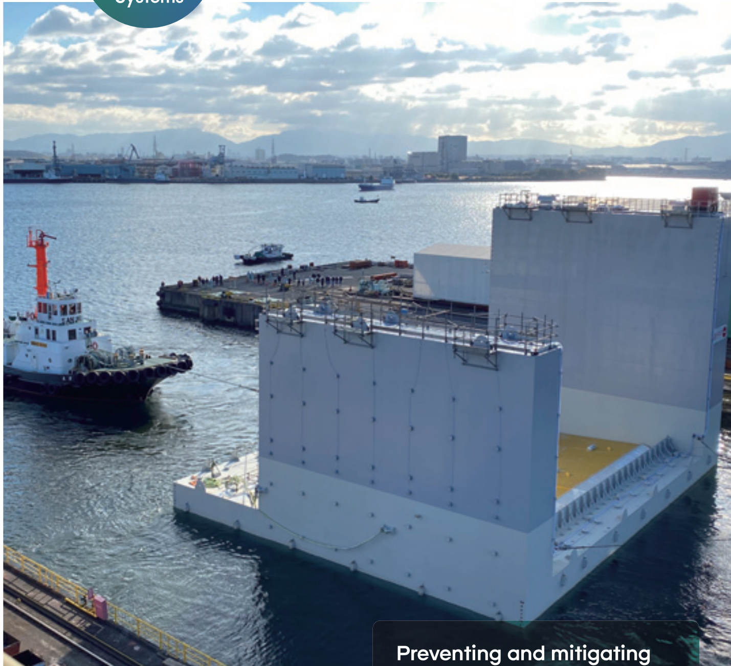
Shield tunneling machines
