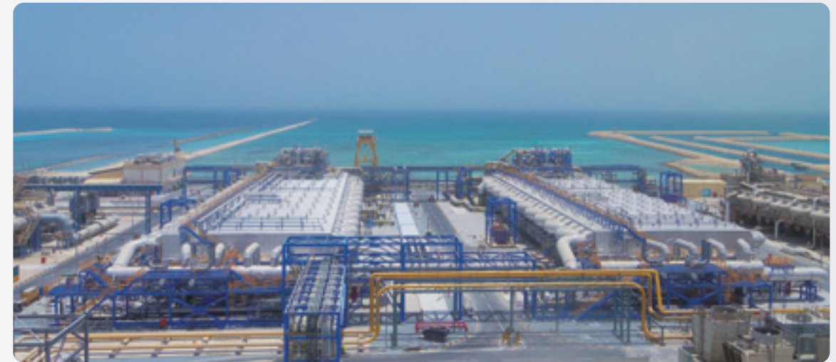
MSF (Multi-Stage Flash) method Desalination Plant (Qatar)
