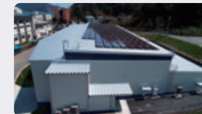
● Control Equipment Center
