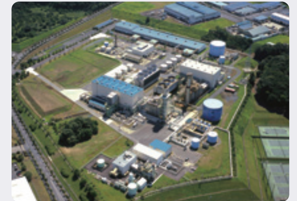
Kanadevia Ibaraki Power Station
