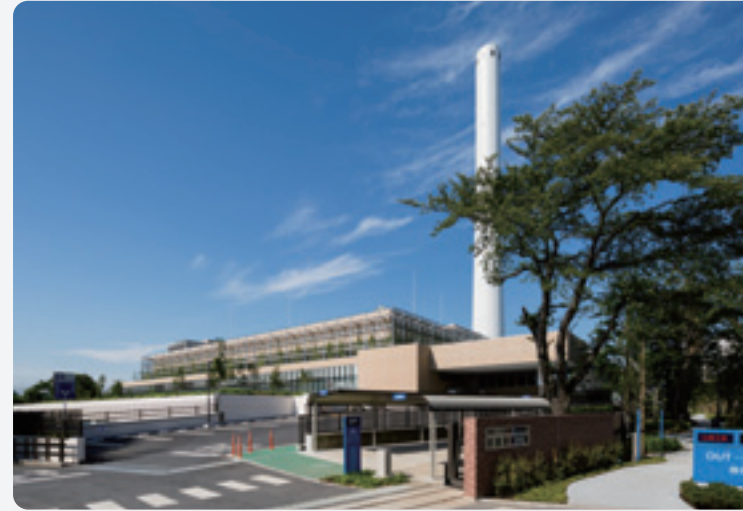
Clean Authority of Tokyo/ Suginami Incineration Plant
