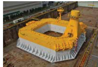
浮体式洋上風力設備 (NEDO 次世代浮体式洋上風力発電システム実証研究 実証機「ひびき」/バージ型浮体構造物) Floating Wind Equipment (NEDO Next-generation Floating Offshore Wind Power Generation System Demonstration & Research Demonstrator "Hibiki"/ Barge-type Floating structure)
