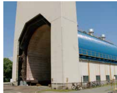
焼鈍炉 Annealing furnace
