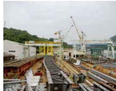
仮組立ヤード Trial Assembly Yard
