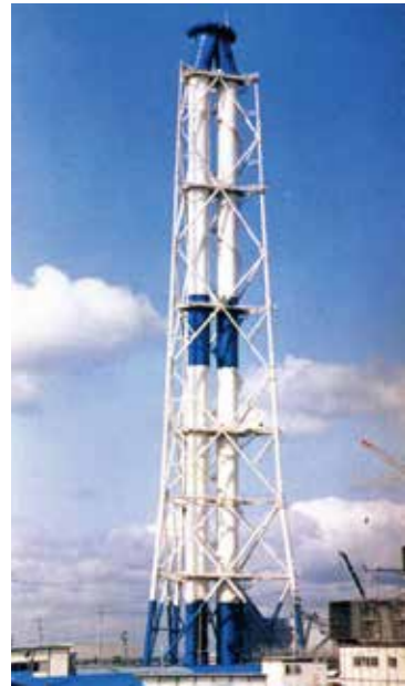
鋼製煙突 Steel Stack
