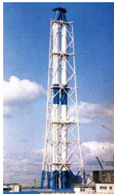
鋼製煙突 Steel Stack
