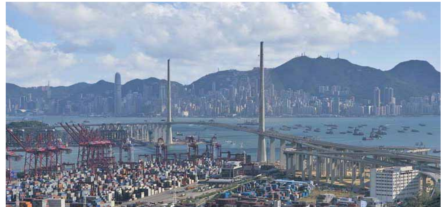
香港・昂船洲大橋 Stonecutters Bridge in Hong Kong
