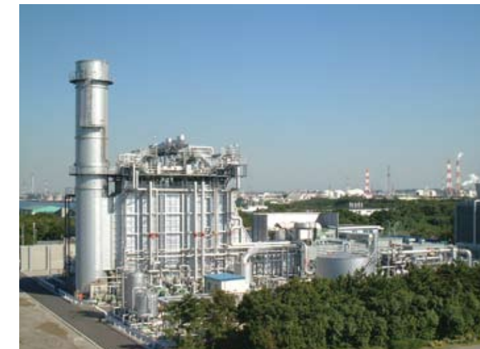
排熱回収ボイラ(横型自然循環式) Heat recovery steam generator (Natural circulation type)
