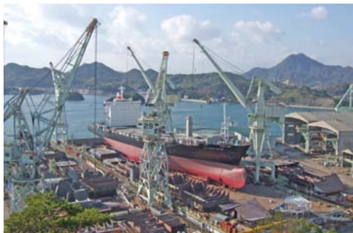
建造中のコンテナ船 (1号船台) Container vessel that is being built (No.1 building berth)
