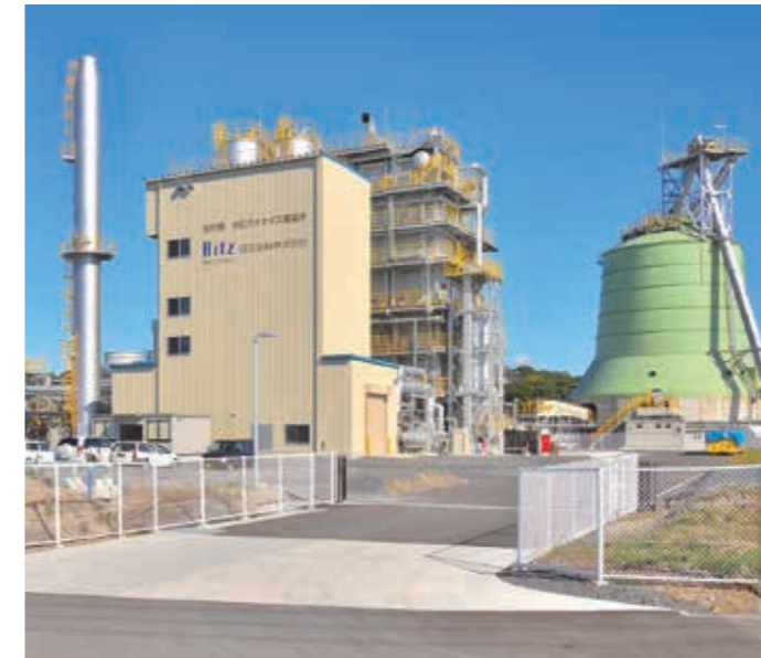
宮の郷発電所全景 Overview of Miyanosato Power Station
