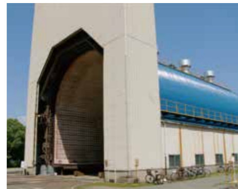
焼鈍炉 Annealing furnace
