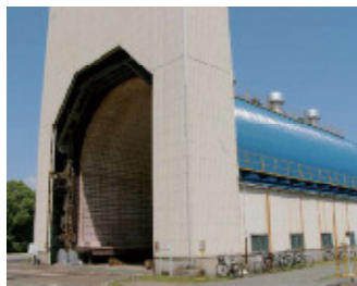
焼鈍炉 Annealing furnace
